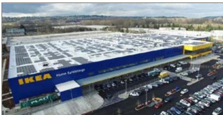
The new store takes into account our environment as it features the state's largest rooftop solar array. The panels, measuring 244,000 square feet, will produce a little over 1.2 million kilowatt hours of electricity annually and remove the equivalent of 187 cars from our roads or provide enough electricity to power 131 homes yearly.
