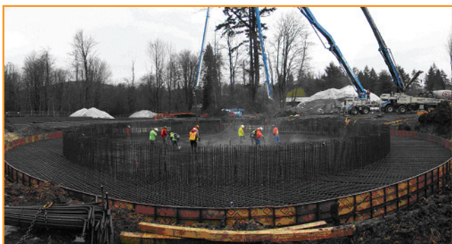
Placement of Reinforced Steel for Reservoir Foundation and Ringwall.
