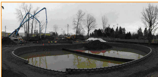
Reservoir Overflow and Stormwater Pond
