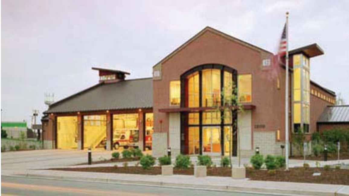
The Fire Station 12, built in the Renton Highlands area
