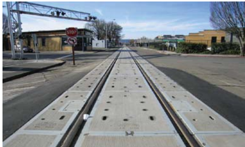
Houser Way South
