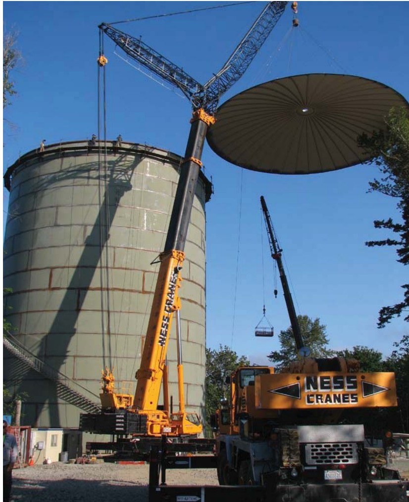
Placement of Roof over New Hazen Reservoir
