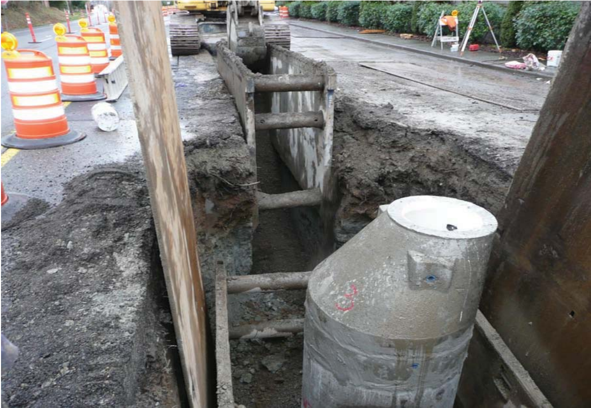
Duvall Sewer Interceptor Installation
