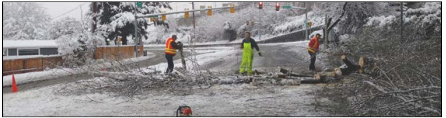
PUBLIC WORKS CREWS CLEAR A DOWNED TREE THAT WAS BLOCKING GRADY WAY
